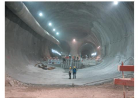
**Above:** The new Gotthard Base Tunnel runs two parallel single-track rail tubes through the Alps.
